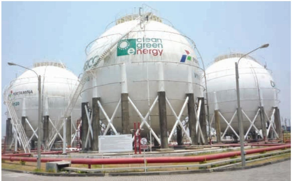
Gambar 2, Tangki Timbun Bulat (Spherical Tanks) di OPSICO
